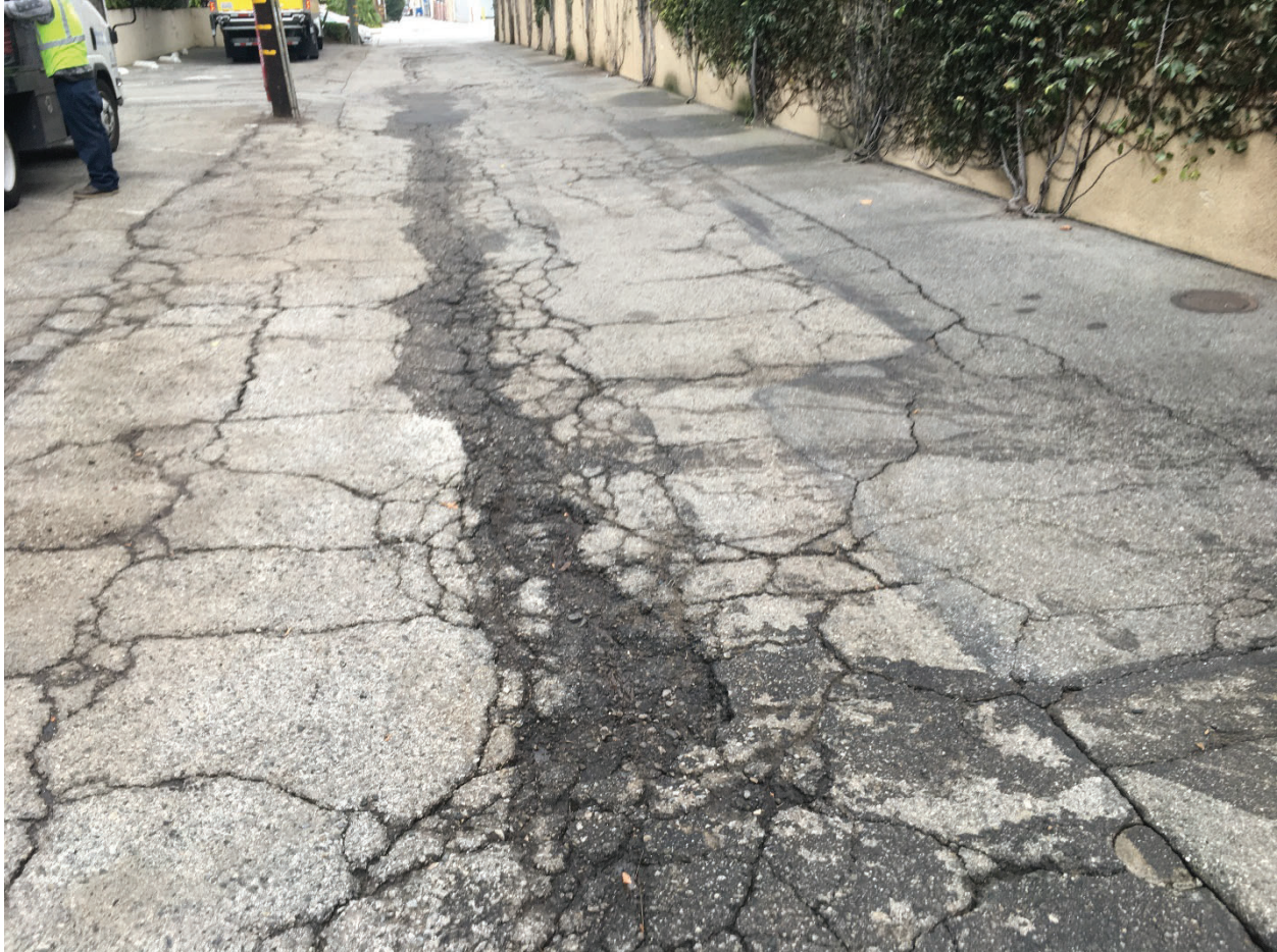
Figure 2. This photo shows the area affected by the leaked fluid. The fluid pooled in the center of the alley and travelled west down the alley. It was reported that the fluid was removed with absorbent material and the ground was steam cleaned. At the time of the photo, there was no oil present. What is seen here is staining. There are no sewer or drainage systems affected. Visual staining was present on the alley surface.
