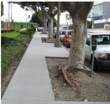
Sidewalk - Enlarged Tree Well.jpg 197K
