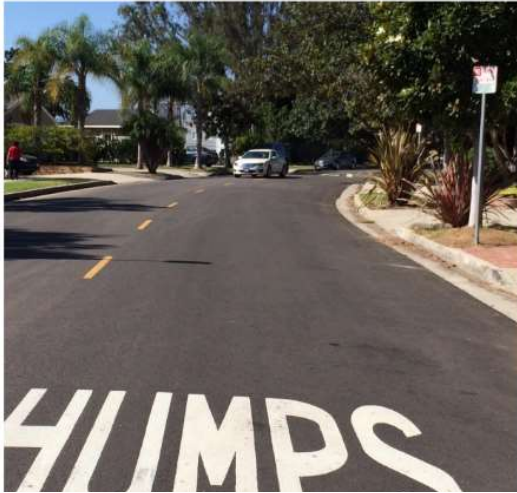
Image for Note 7: The speed hump at the top of this image is visible from the “HUMPS” marking at approximately 200 feet away
